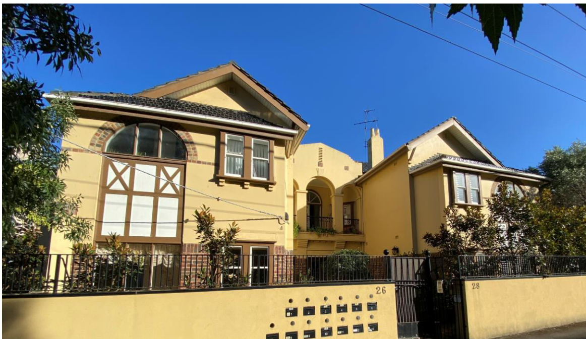
X-pattern Tudor Revival half-timbering, with Arts & Crafts brick arches and clinker bricks.
