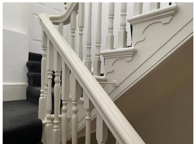
The spiral handrail end and the turned timber balusters are typical of Victorian era stairs.
