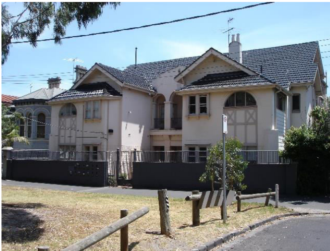
In 2009-10, after the birch trees were removed.
